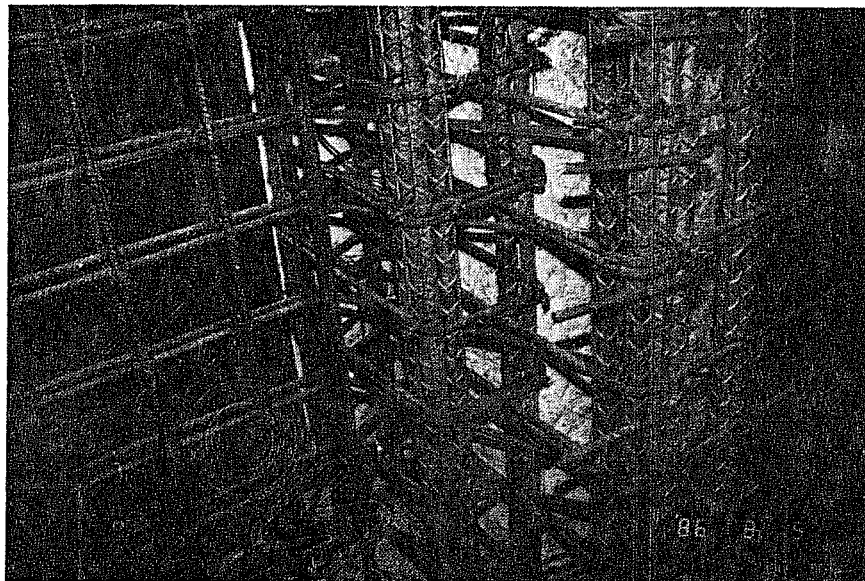
Figure 1.4 Column Jacketing Using Bundled Bars
